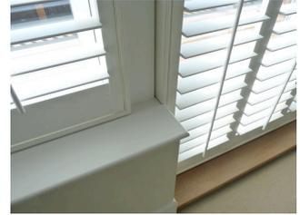
Replace the insert strips into the frame to cover the screw heads.
