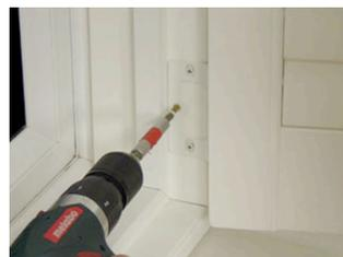
Check you have enough window frame to screw into, you may need to re-drill your own pilot holes at an angle or in line with a window mullion to ensure they have something to fix into, if possible use a long extension bit to ensure the chuck of the drill does not mark the wall.
