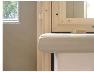
When there is no infill, screw the 3 frames together.
