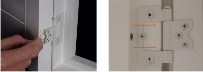
Hinge packers are provided to help line up the shutters within the frames. If you have an out of level window and you need to fit your frame slightly out of level to get the best look, use hinge packers to pack out the panels to help align them.
