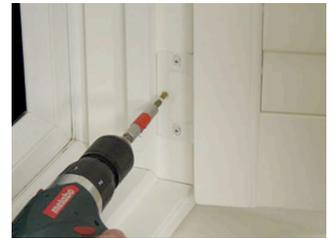
Check you have enough door frame to screw into, you may need to re-drill your own pilot holes at an angle or in line with a door mullion to ensure they have something to fix into.
