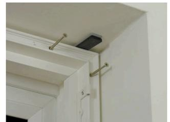
Place 2 or 3 small wedges on the floor depending on the width. Carefully lift the frame into the recess and sit it down on the wedges. Use the rest of the wedges in each corner at the top. Centralise the frame by adjusting the wedges in or out and moving the frame until it looks visually central.
