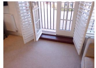
Replace the insert strips into the frame and Tposts to cover the screw heads.
