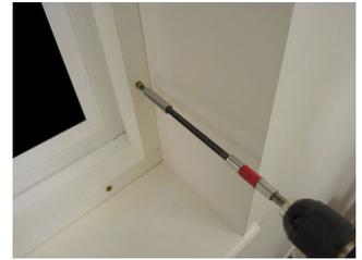
Use a 4-5mm drill and counter sink the holes if possible, especially if you are fixing into UPVC. The number of fixings you use will be dictated by the width of your door, usually 5 holes, 1 x left, 3 x middle and 1 x right.
