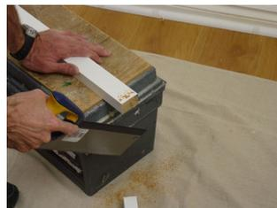
**Battens all round** - measure the bottom width, mark your batten to length, repeat for the top batten. Draw a square line on the top (40mm face) and down the side (30mm face) of the batten to help cut in a straight line, a tenon saw or fine toothed saw is best.
