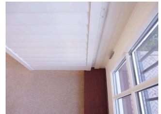
If you want the vertical batten to line up with your Tposts, then consider fitting this behind the shutter frame once it's been fitted, being able to do this will depend on the design of doors and how much room you have.
