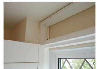
Tposts can be screwed to the door frame just like the outer frames. Not all Tposts have inserts, so some types can not be fixed they are just held in place by the top and bottom screws.
