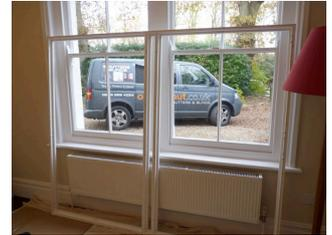
Tposts are an extra part of the frame that need to be screwed into place before you fit the shutters.
