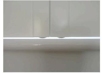
If you have clamped the frame into position, lift the left set of shutters into place first. Adjust the frame and shutters so there is an even clearance gap between the shutter and frame all round. A small wedge on the window sill can be used to help support the shutters and hold them in the correct position.
