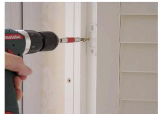
Before finishing the rest of the fixing, ensure the shutters open and close correctly and that they line up neatly with each other and within the frame. You may need to loosen the frame screws to make any adjustments. If more extreme adjustments are needed, remove the screw and re-drill a new pilot hole.
