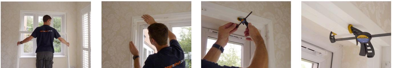
Carefully lift the frame into position. (This example uses a 3 sided design.) Line up the frame, check it's level and to make it easier to fit if you are on your own, use a small clamp to hold the frame in place.
