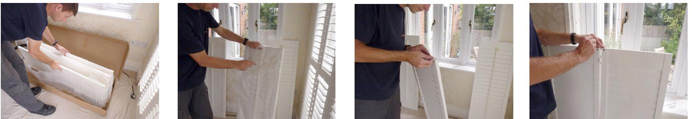
Unpack the shutters, the mouse hole (where the control rod fits) will indicate the top of the shutters. If you have the hidden tilt rod, the top rail should have the small rebate facing you, the bottom rail rebate should be at the rear of the shutter.
