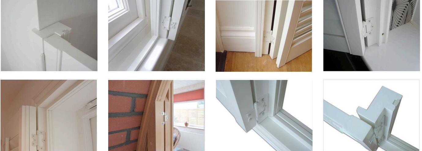
When side fixing a Z frame you do not need any rear battens. The frame can be screwed sideways and the fixings are hidden by the removable insert strips.
