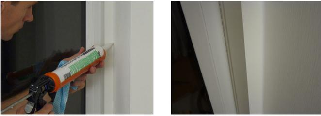
Use decorators filler (Caulk) in a tube, for example 'No Nonsense' from Screwfix is suitable.
