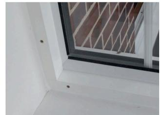
Choose to fix the battens into the window or down into the window will. Use a 4-5mm drill and counter sink the holes if possible, especially if you are fixing into UPVC. Drill the pilot holes in the battens where you marked them and fix the top and bottom battens in place.
