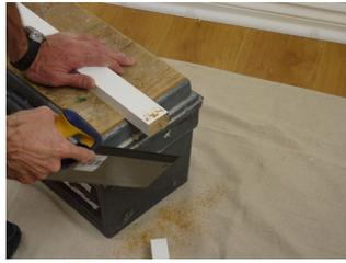
Measure the width of the centre bay at the top and bottom, the battens should run the whole the length of the window. Draw a square line on the top (40mm face) and down the side (30mm face) of the batten to help cut in a straight line. A tenon saw or fine toothed saw is best.
